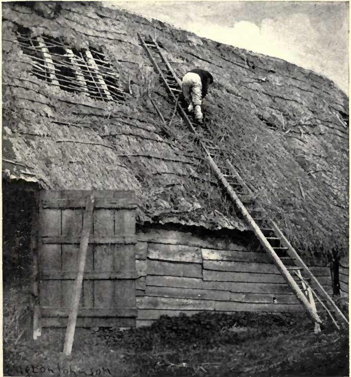
Patching the Thatch Roof of a Barn
